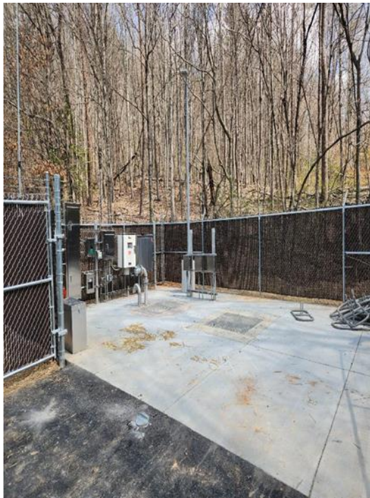
(Brushy Valley Lift Station upgrades)
