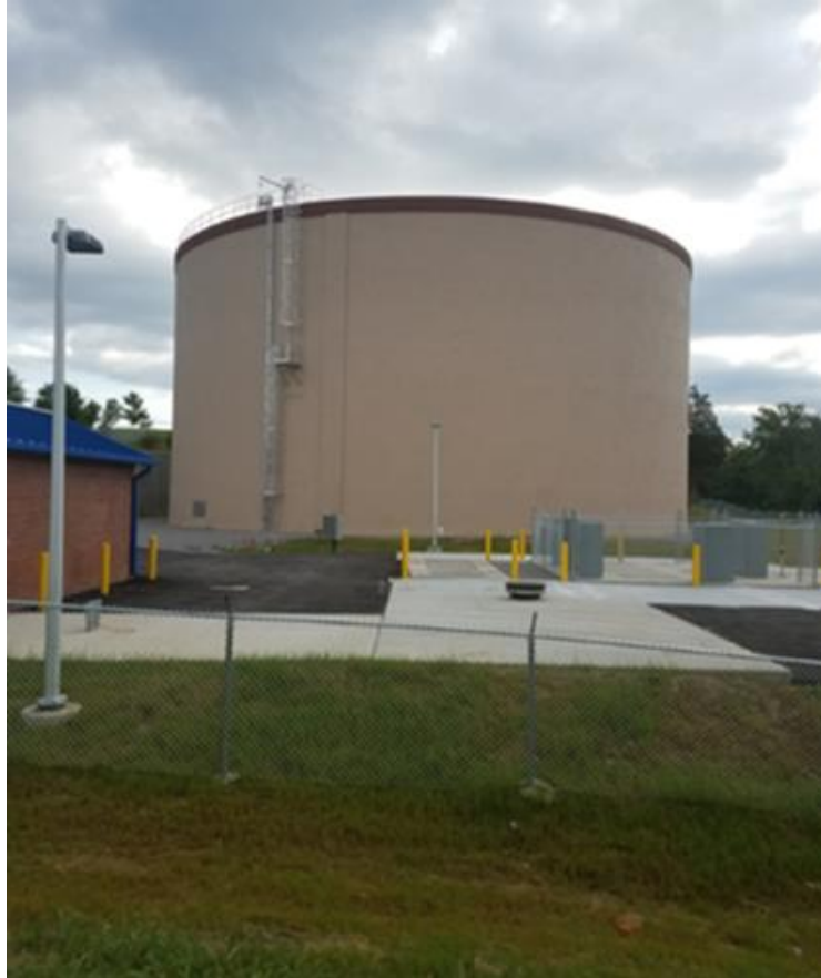
(Dry Gap Pike storage tank & lift station)
