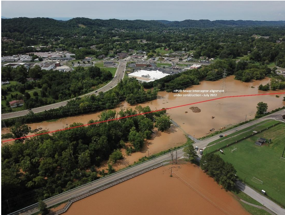
July 2022 Flooding along Beaver Creek – The red line shows HPUD’s sewer interceptor alignment that was under construction at the time.
