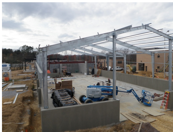
Structural Steel for Covered Storage Pad
