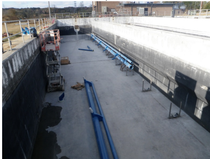
New Jet Aeration Piping in Digester #5
