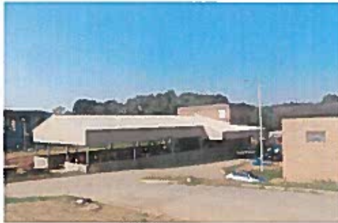
New Covered Sludge Storage Pad
